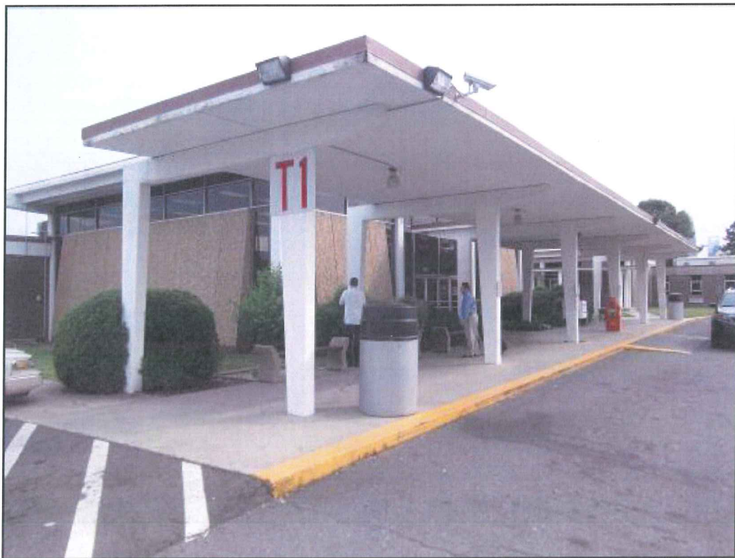
Figure 15: View of the east elevation and north elevation extended canopy
