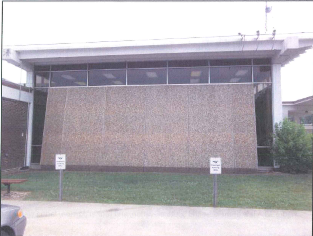
Figure 16: View of the east elevation, northern block, facing west
