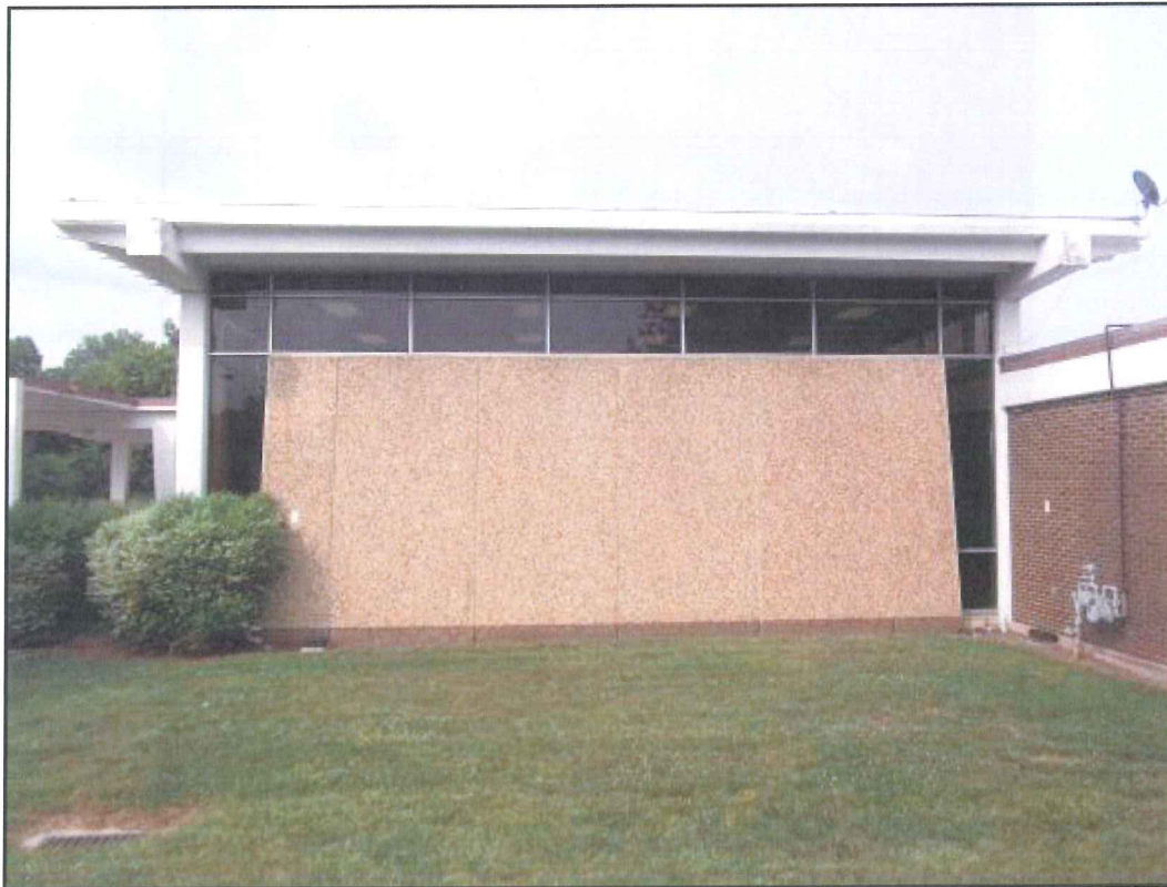
Figure 11: View of the west elevation, northern block, facing east
