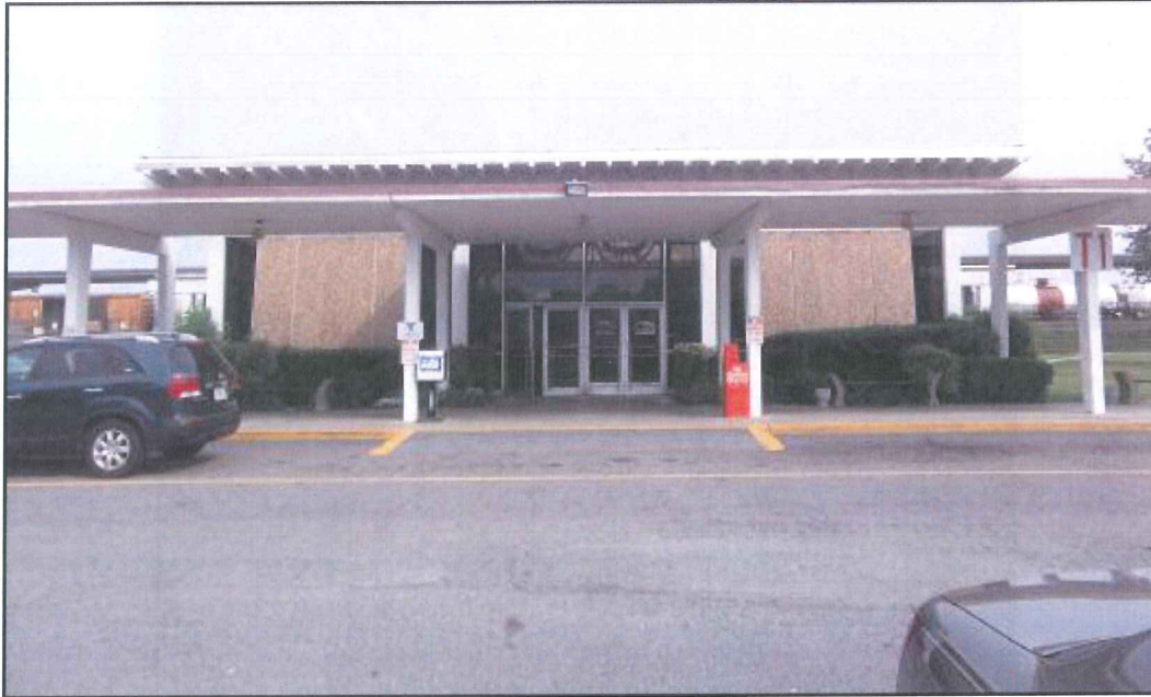
Figure 10: View of the north elevation, facing south
